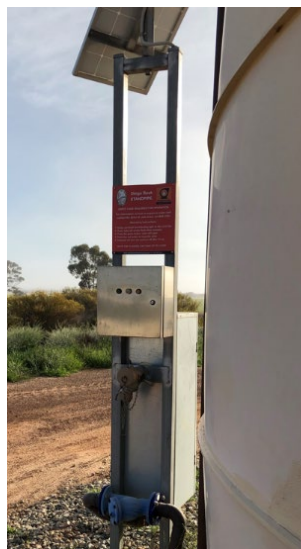
Swipe card standpipe system
