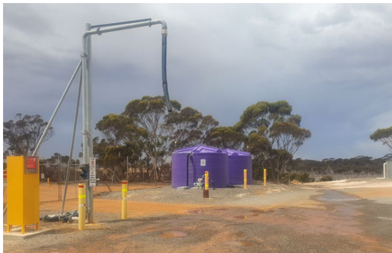
Standpipe and swipe card system (February 2020)
